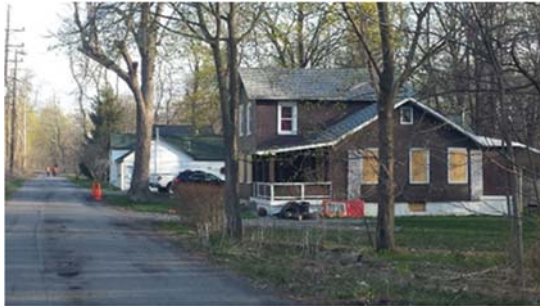
Above: Homes on Water Street prior to demolition
