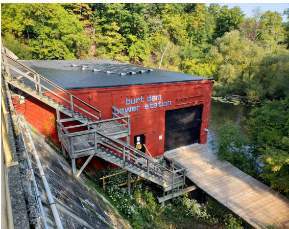
Below: Burt Dam power station September 2020
